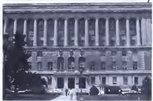
South Office Building, south elevation.
